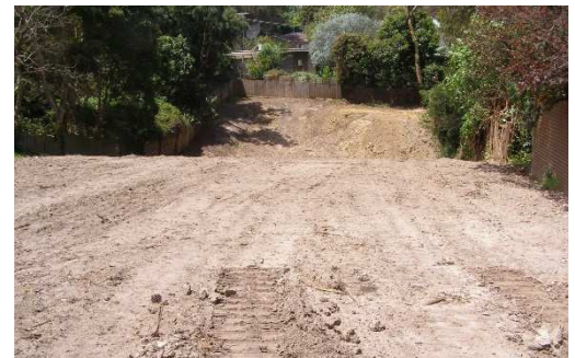
Vegetation cleared for building redevelopment.
