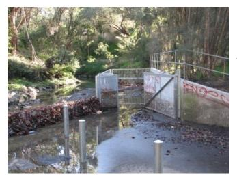
Work on the replacement of the litter trap just upstream of Blackburn Road has been completed. The new litter trap is not working as expected due to large numbers of deciduous leaves getting caught in the vanes. Melbourne Water has planted several plants on the banks adjacent to the trap. We hope to find out more about their plans for revegetation at our August meeting.
