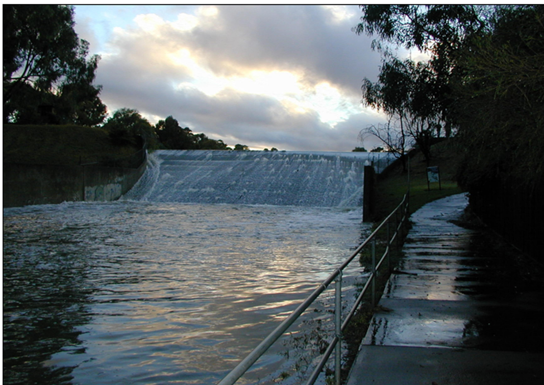
Water overtopping the Mount Waverley Wetlands Dam in 2005
