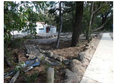
Drainage works - View from Wills Ave looking SW
